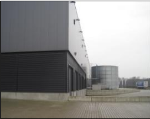
Loading dock zonder dockshelter
